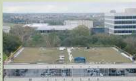
Building 12 at JSC under construction in Houston, Texas.
